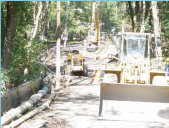
Mill Creek Sewer Replacement
