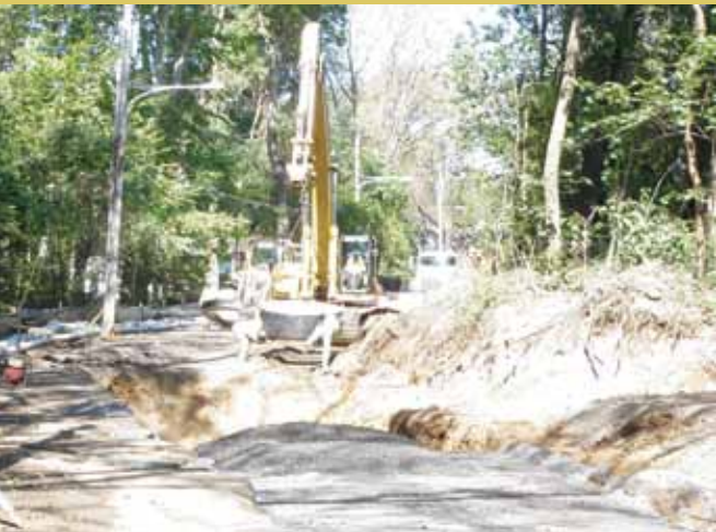
Mill Creek Sewer Replacement
